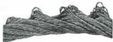
12. Strand core protrusion as a result of torsional unbalance created by 'drop ball' application. (i.e. shock loading).
