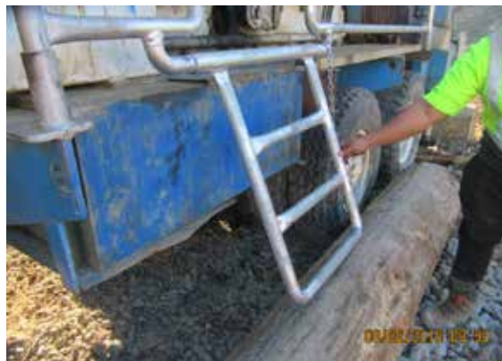
Improved access with integral ladder. Needs kickplates added and something better than the de-barked log as a lower step.
