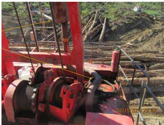
Unguarded potentially hot exhaust and muffler adjacent to access ladder.
