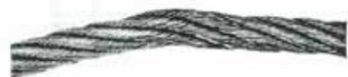
13. Typical example of localised wear and deformation created at a previously kinked portion of rope.
